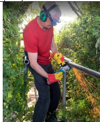
Peter fettled the existing handrails and remounted the ends making a very neat job.
