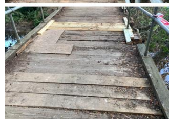
Both sets of three timbers we've installed. Still waiting for BC PRoW team to get quotes for complete replacement.
