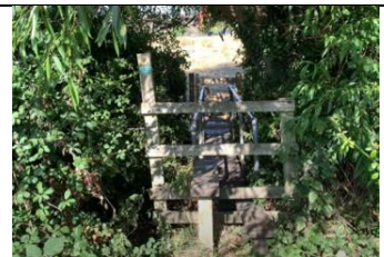
The handrails were reduced in length and finished off nicely using the existing kee-clamp fittings.
