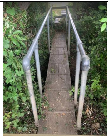
The handrails were reduced in length and finished off nicely using the existing kee-clamp fittings.
