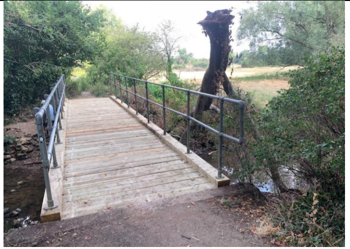
1/8/26 Haddenham HAD/2435 on HAD/17/1 at SP738074 following rebuild by BC contractor.
