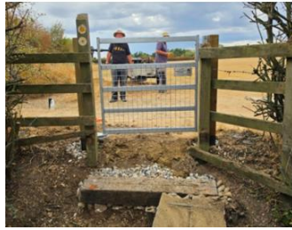
Gate 395 - Half-sleeper used to great effect to improve passage through newly installed gate.
